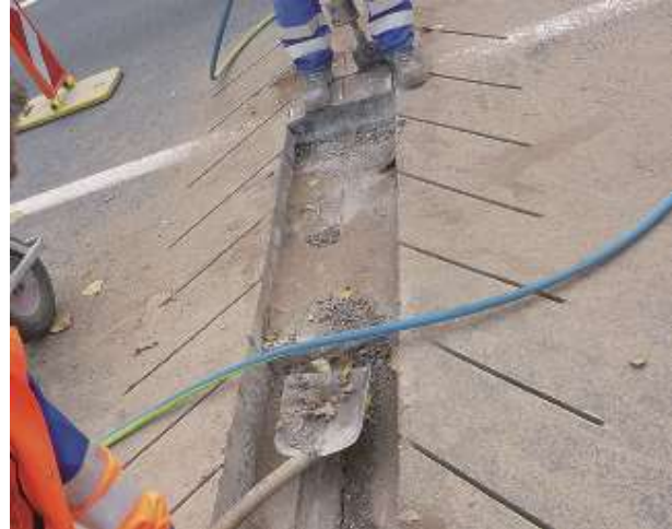
Removal of existing joint / surfacing as required
