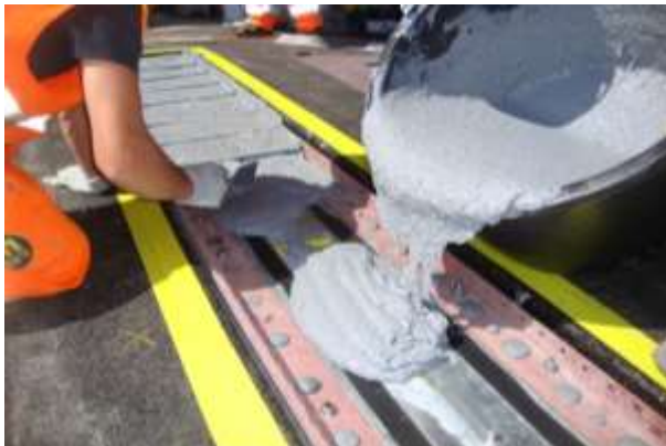
Placing of PU material
