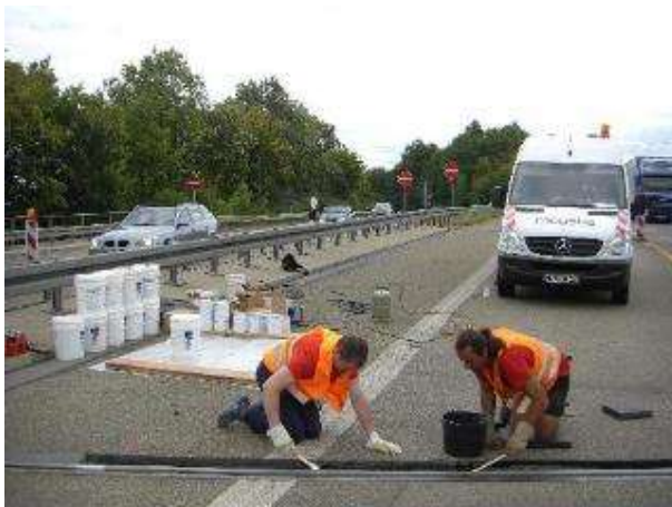
Application of primer to substructure
