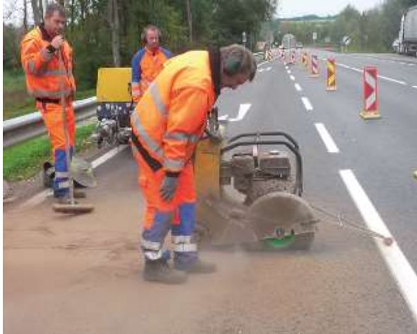
Cutting of continuous surfacing across the joint
