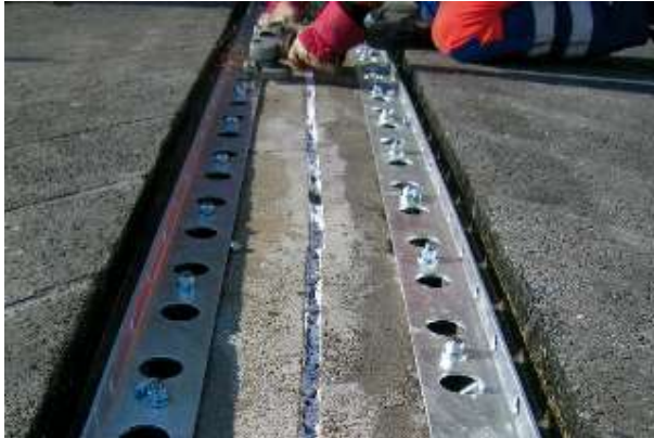
Fixing of steel angles to polymer concrete base
