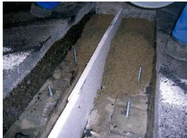
Forming polymer concrete base (Styrofoam in gap)
