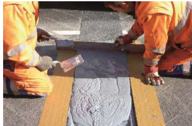
Precise levelling of material to connecting surfaces
