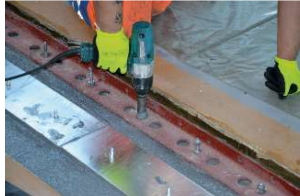
Fixing of steel angles, and coverplate across gap
