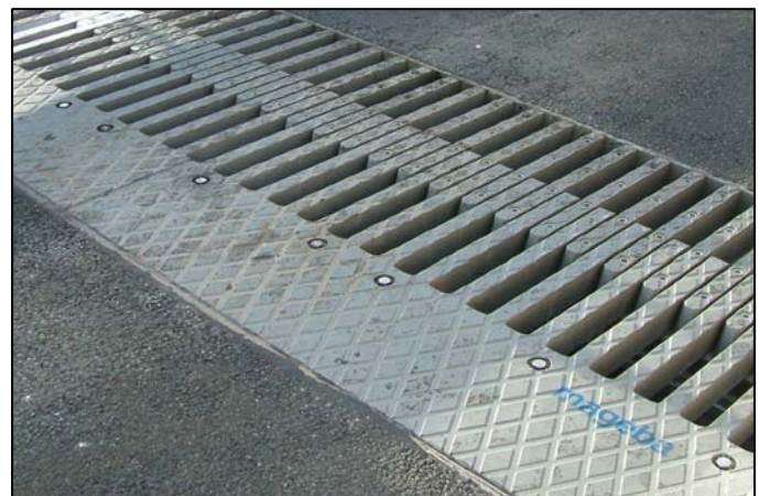
Figure 4: Sliding finger joint (Steel system) – As installed
