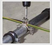
Simply strip some insulation from the earthing wire, insert the wire from the side and tighten the contact screws.
