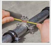
Easy installation of equipotential equalization without interruption of the potential equalisation conductor.
