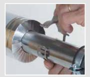
Place the equipotential bonding and earthing clamp around the metal pipe ...
