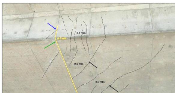
Figure 10. Cracking of concrete on underside of deck at coupling joint of cables
