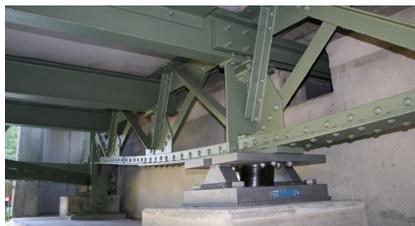
Seismic damper in access shaft, from above (connecting through wall on right to deck girder)
