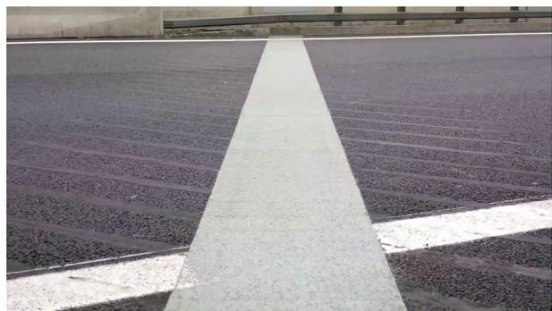
Figure 7. Modern flexible plug expansion joints of polyurethane (PU) offer far better performance and durability than the traditional asphaltic type
