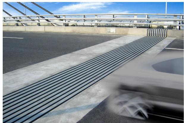
Figure 1. The modular expansion joint divides a bridge movement gap into a number of small gaps
