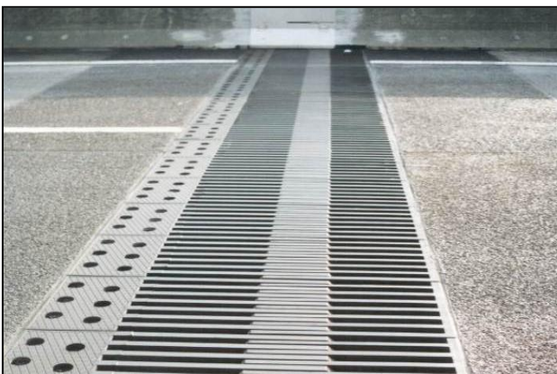
Fig. 3: An installed Tensa-Flex expansion joint
