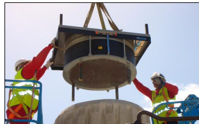
Fig. 12: Installation of an elastomeric bearing on site, showing the stainless steel sheet on top which allows longitudinal sliding movements
