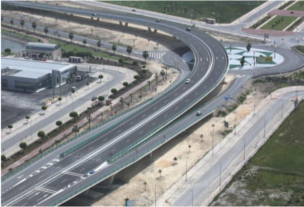
Fig. 1: The Viaducto Puerto de Santa Maria – aerial view showing the structure's curve
