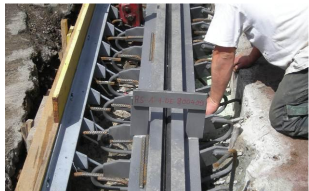
Fig. 9: Use of a joint requiring anchorage in normal concrete is far less convenient when installed to replace an existing joint
