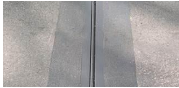
Fig. 14: A hump seal fills out the gap, keeping it clean, reducing noise under traffic and increasing pedestrian comfort
