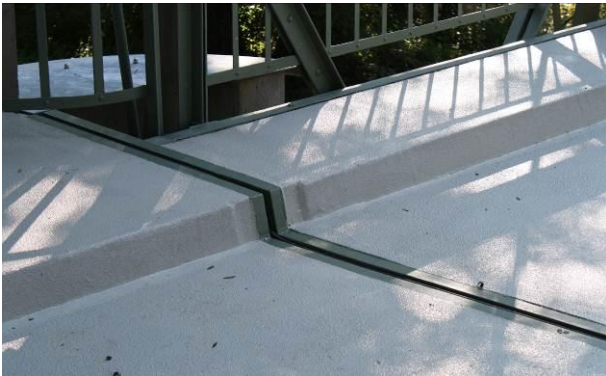
Fig. 2: A typical single gap joint, consisting of well-anchored steel edge profiles connected by an elastomeric strip seal
