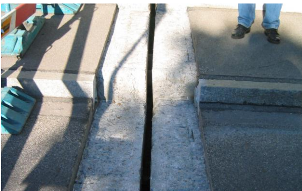
Fig. 8: The anchorage in polymer concrete minimises break-out – often requiring only removal of the old joint and asphalt surfacing
