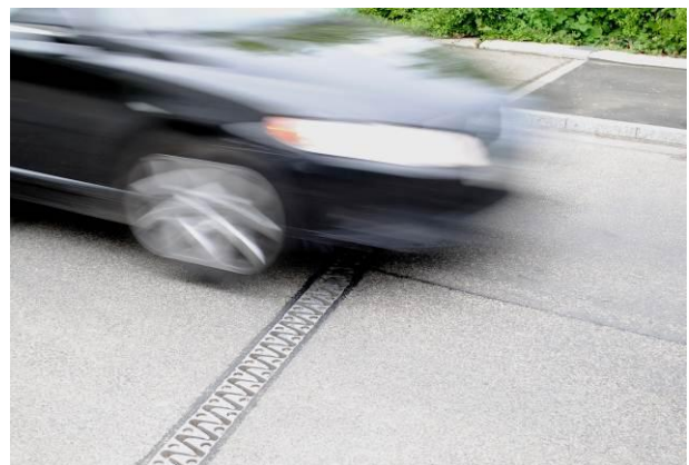
Fig. 1: Small movement expansion joint (single gap joint with noise-reducing surface plates)
