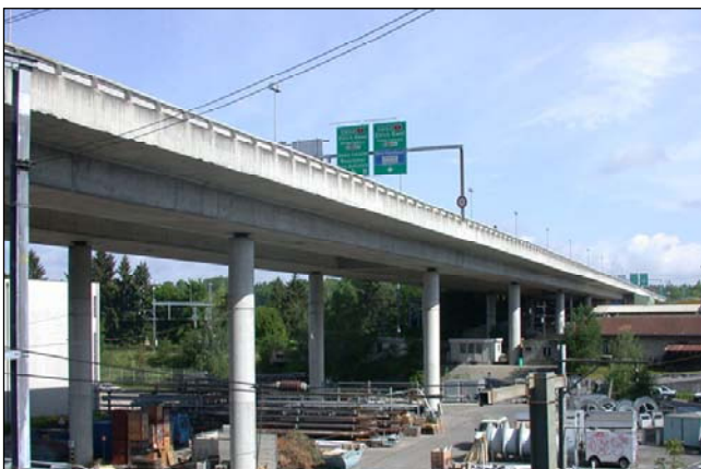
Fig. 1: Weyermannshaus Viaduct, Berne - Switzerland
