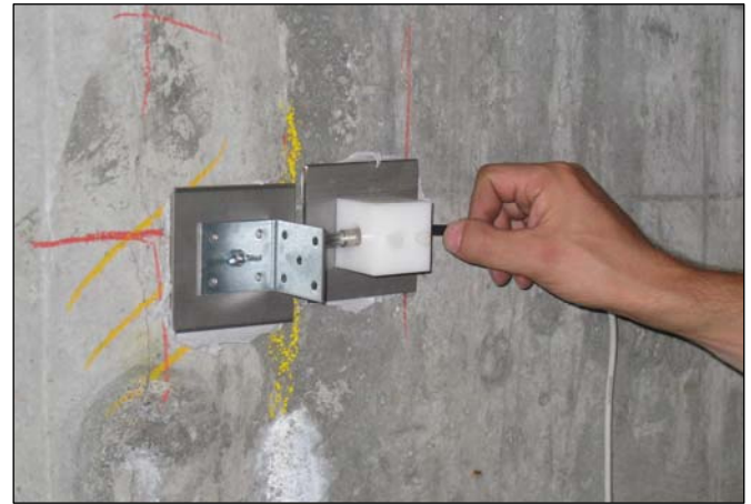
Fig. 5: Installation of an inductive sensor
