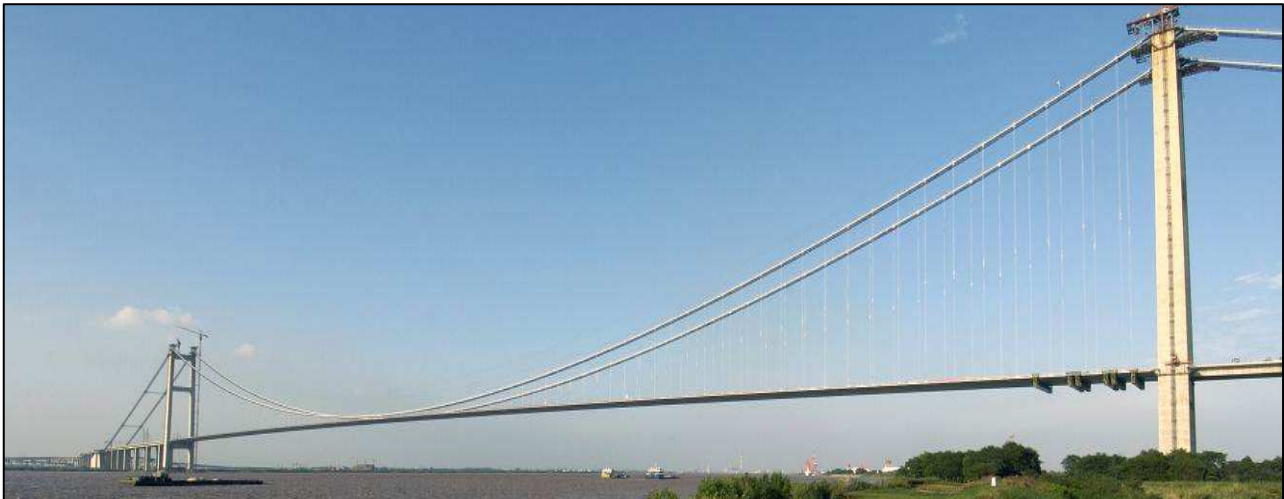
Fig. 8: The Run Yang Yangtze River Bridge in China, with its 1,490m main span – equipped with 27-gap modular joints since constructed in 2004 (world record joints at the time)
