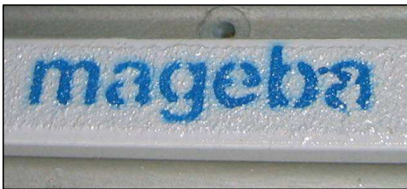
Fig. 7: Anti-skid surfacing on the driving surface of a modular joint's lamella beam
