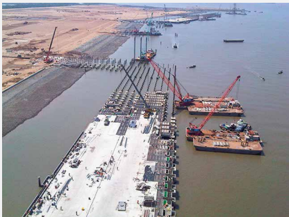
New construction of Cai Mep deep-water port, Vietnam
