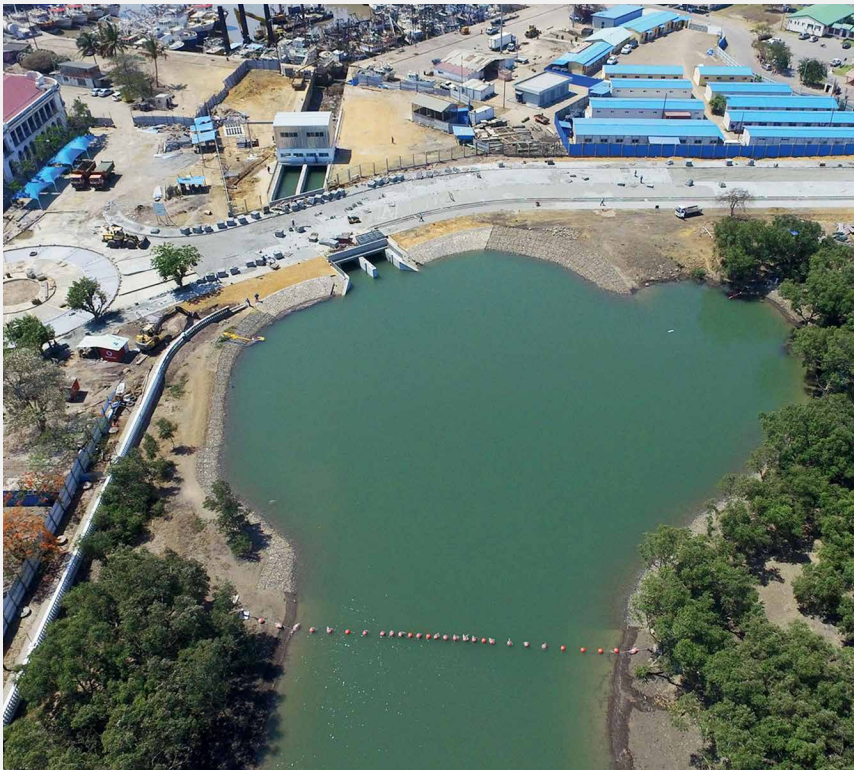
Beira flood barrier, Mozambique
