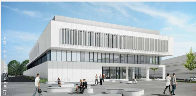
Max Planck Institute for the Structure and Dynamics of Matter, Hamburg (in progress)
