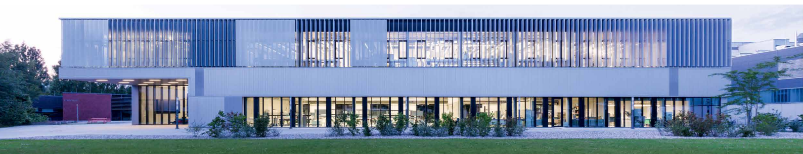
Institute of Civil Engineering, Faculty of Engineering / © Wismar University
