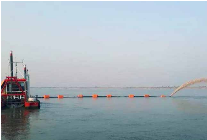
Dredger in action on the Ganges River
