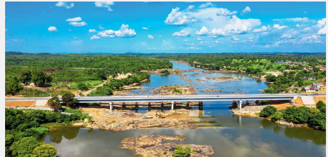
Bridge over the Sewa River, Sierra Leone
