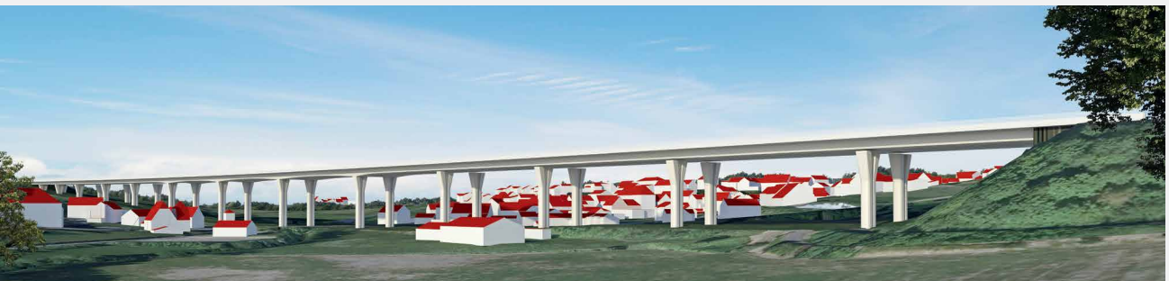
Utrichshausen Valley Bridge on A7 autobahn (preferred option showing ground modelling and the city in the background), DEGES, Hessen, Germany
