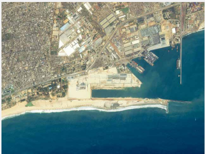
Phased expansion of Lomé deep-water port, Togo
