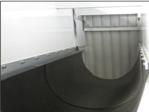
Fig. 11: Robo ® Silent noise insulation beneath an expansion joint (fully installed)
