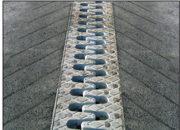
Fig. 12: Robo ® Dur reinforcing ribs in asphalt adjacent to an expansion joint
