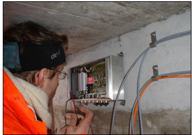
Figure 7: Wiring of central computer
