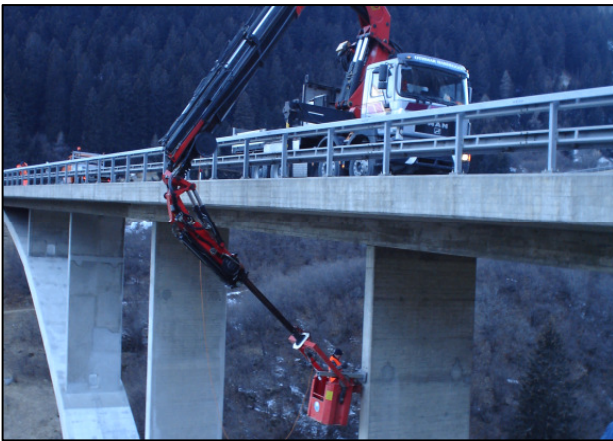
Figure 6: Installation of a solar panel
