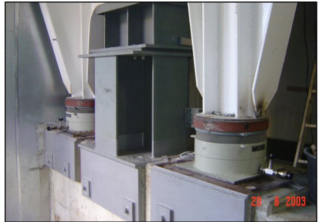
Figure 13: Regulation of bearing height
