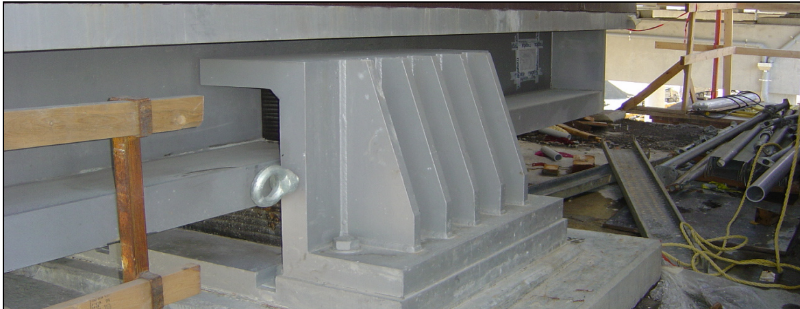
Fig. 7: Installation of a bridge bearing
