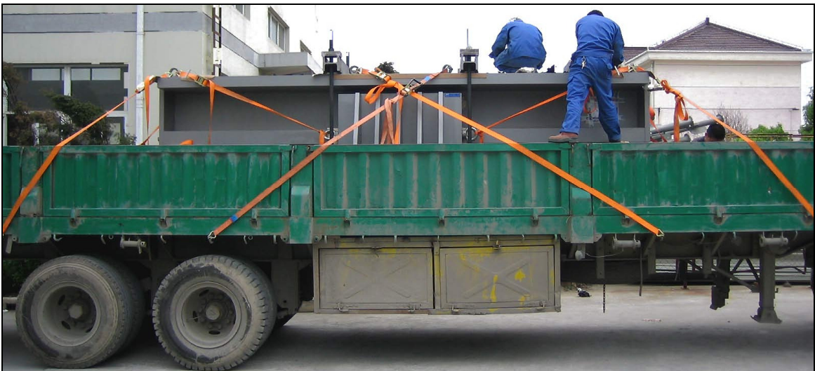
Fig. 6: One bearing being secured on a lorry for transport to site
