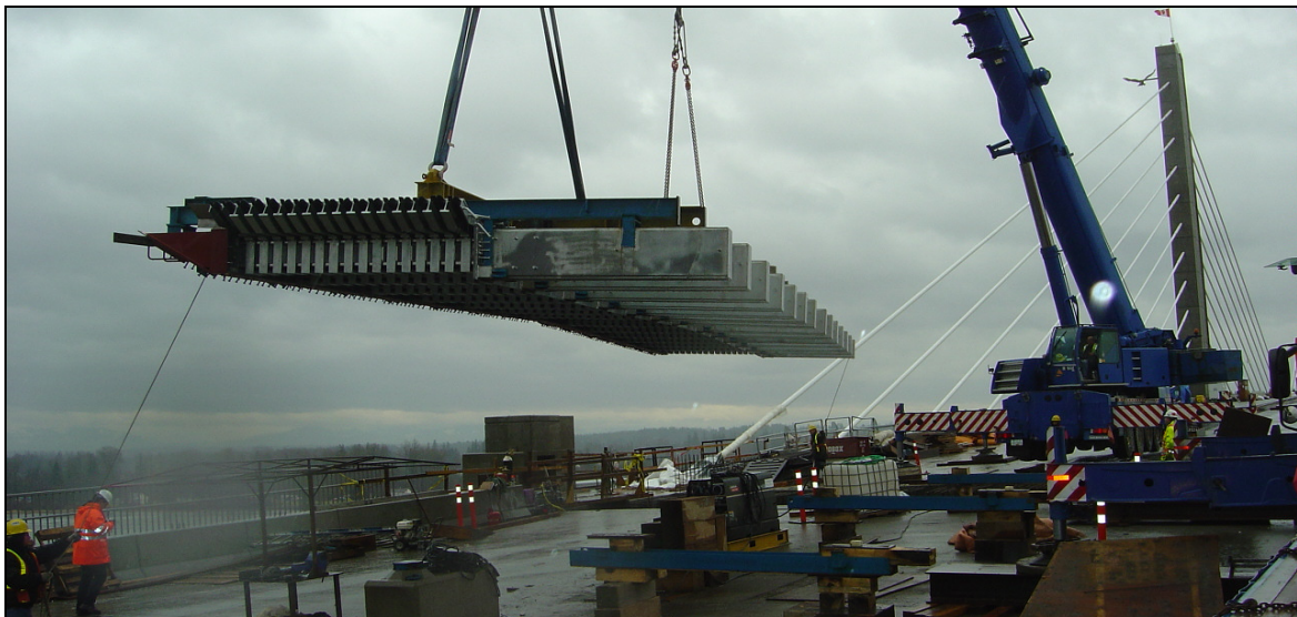
Fig. 10: Lifting in of one mageba LR17 expansion joint of length 24.5m
