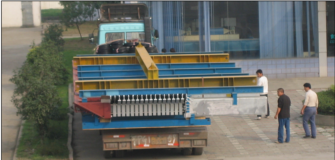
Fig. 9: Expansion joint with Fuse-Box (at left side) ready for transportation
