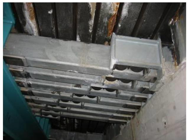
Figure 1 - Multiple support bar system (1970)
