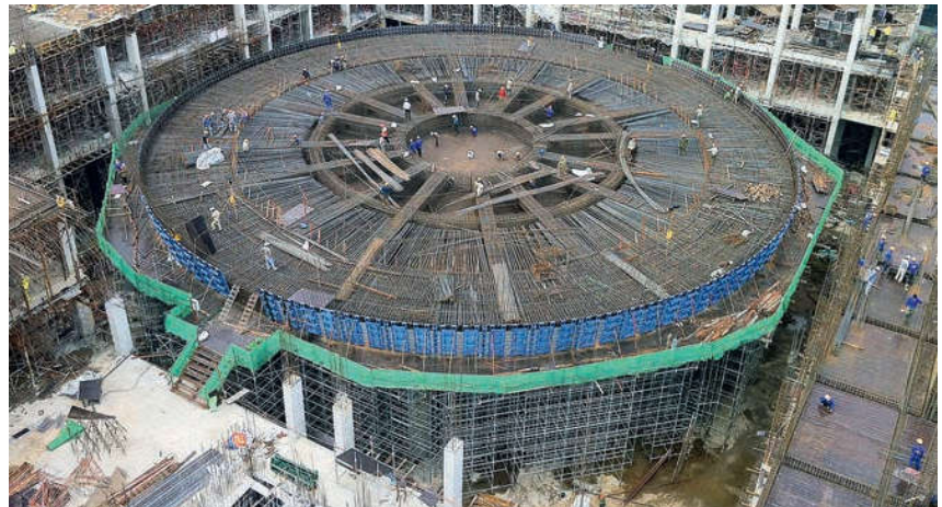
Construction of the Main Meeting Hall's base slab
