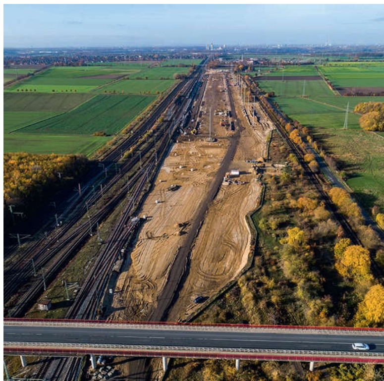
Overview of construction site
