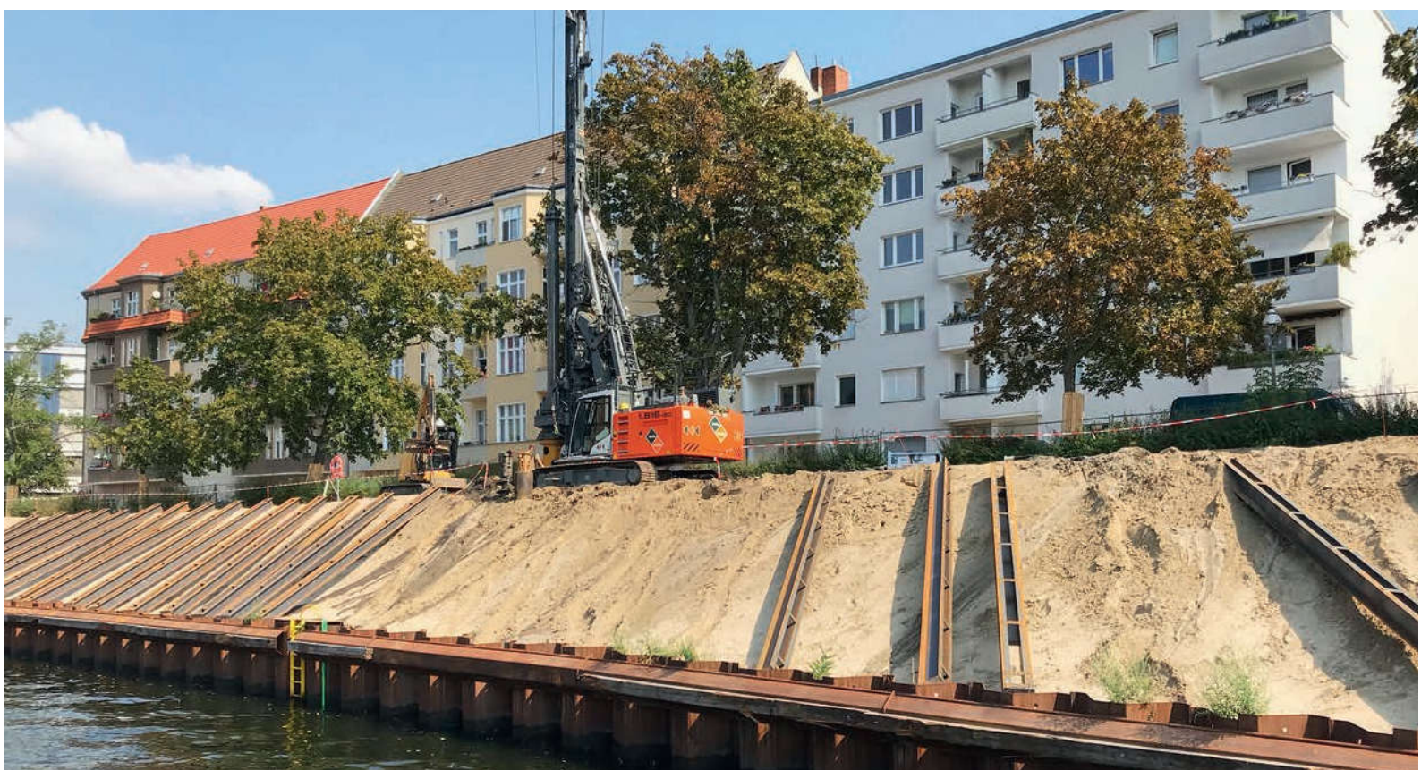
Installation of sheet piling on the Viking Bank
