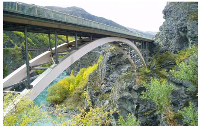
Figure 11. The monitored bridge, crossing a valley
