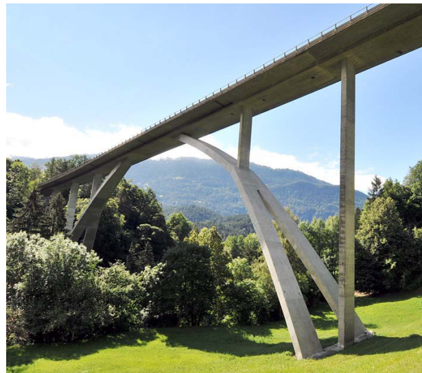
Figure 6. The Lavoitobel Bridge, Switzerland
