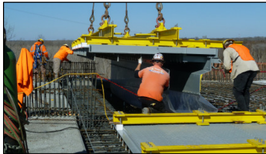
Figure 20. Lifting into position of the second expansion joint at Axis 3E.
