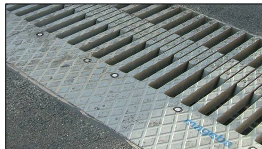
Figure 8. Sliding finger joint (steel system) – As installed.
