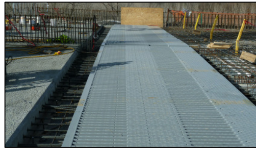
Figure 21. Axis 3E following positioning of both its expansion joints
