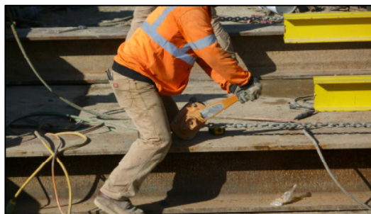
Figure 14. Opening of joint (adjustment of pre-setting).
