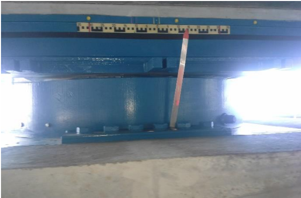
Figure 26. A bearing as installed, before final application of dust skirt to protect sliding surfaces
