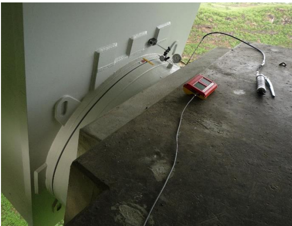
Figure 9. The injection method can be used with suitably designed Reston-Pot bearings in any situation, e.g. to adjust distribution of loads among the bearings of an arch bridge
