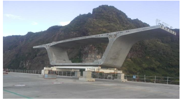
Figure 3. A precast segment of the box girder bridge, ready for connection to the end of the extending superstructure
