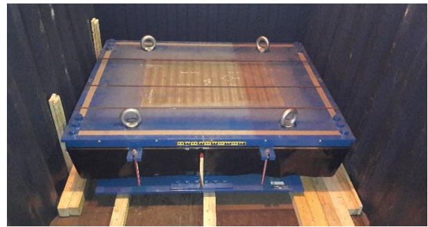
Figure 24. Transportation of bearings to site in shipping containers for maximum protection from damage during transit
