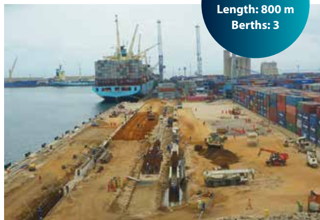
Quay construction phase
