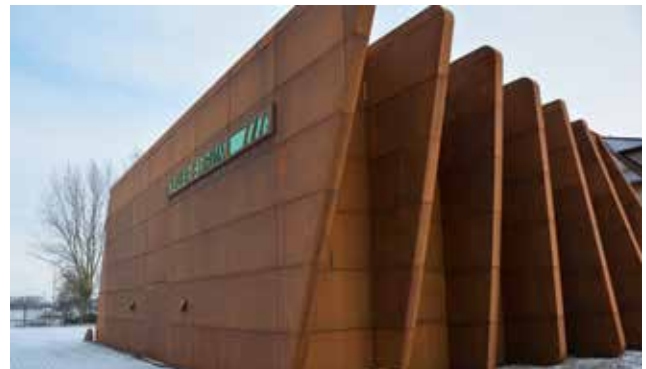
Onshore power supply building
