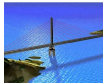
Agin Bridge (TR)
