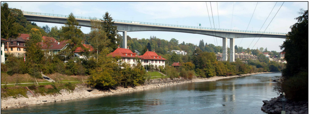
Figure 5: Felsenau Viaduct, Bern
