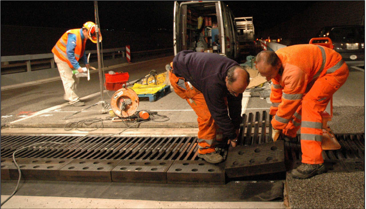
Figure 6: Night-time installation of the Tensa® Flex Sliding Finger
