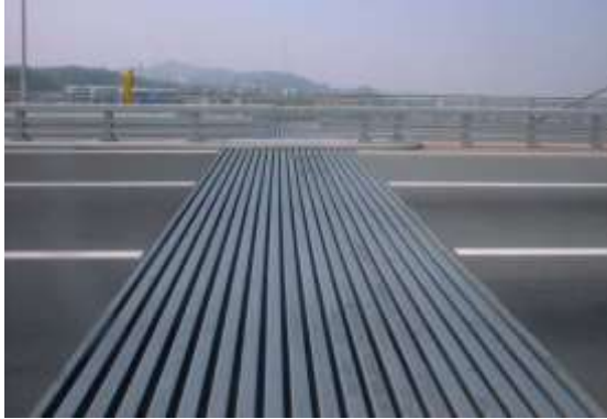
Figure 1. A modular expansion joint, viewed from above, showing the centerbeams and edgebeams that form its driving surface.
