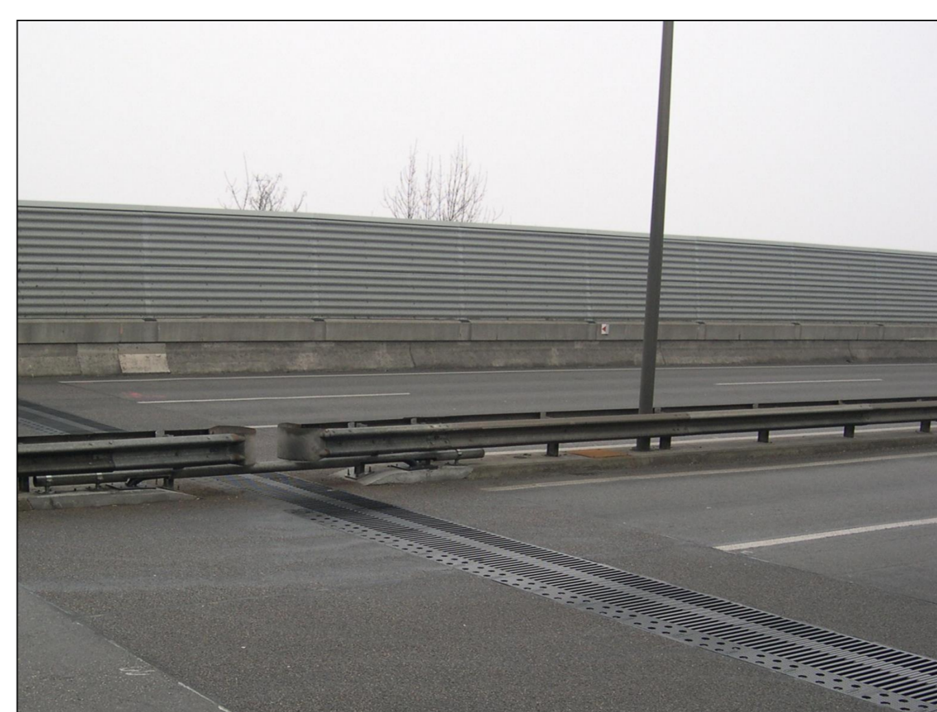
The joint of the Felsenau Viaduct after replacement had been completed
