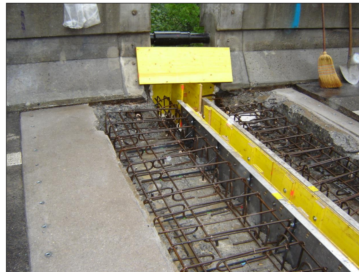
Step 3: Reinforcement was then placed (also during the weekend)
