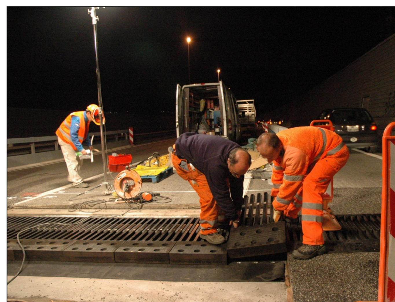
Step 7: On the last night shift, the Tensa®Flex joint was installed
