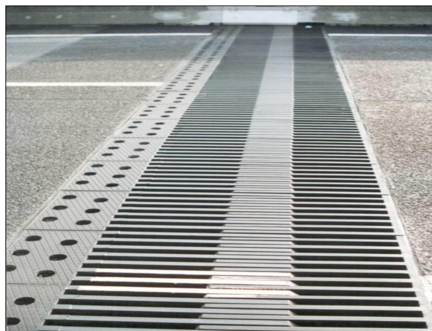
Installed Tensa®Flex Sliding Finger joint
