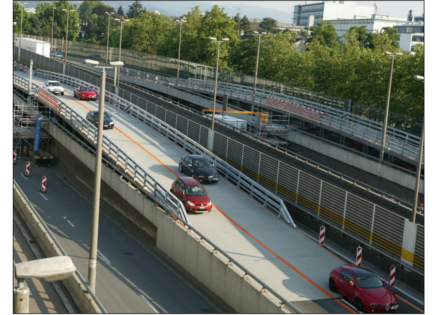
Large fly-overs can be used to keep traffic moving during replacement works
