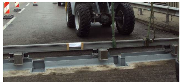
Figure 9. Lifting in of the new replacement part, consisting of centerbeam(s) and support bars etc., complete with “boxes” on ends of support bars
