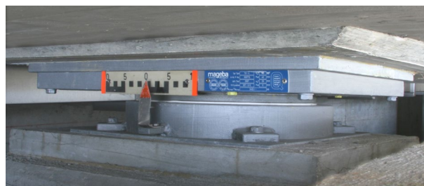
Figure 12. Once installed, a bearing with anchor plates can be unscrewed and removed with only minimal lifting of the superstructure required
