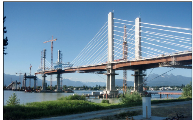
Fig. 7: The Golden Ears Bridge during construction
