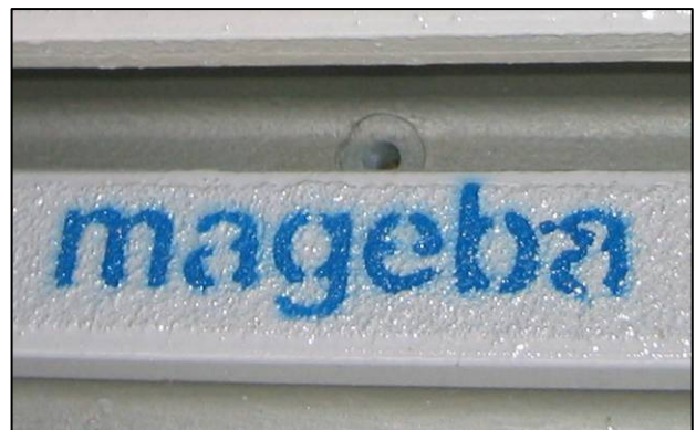
Fig. 5: Lamella surfaced with anti-skid coating
