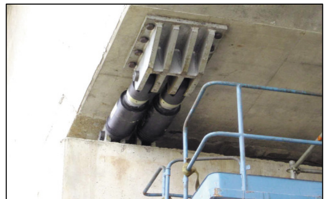
Fig. 16: A pair of shock transmission units
