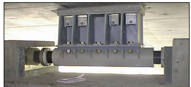
Fig. 14: A preloaded spring damper
