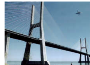
Vasco da Gama Bridge, Portugal
