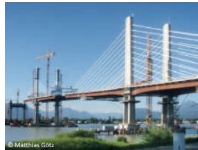
Golden Ears Bridge, Canada
