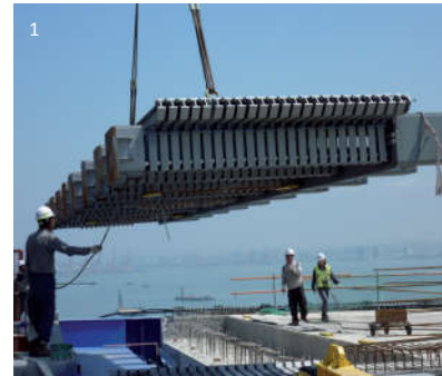
Sliding finger joint
