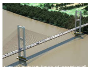
Audubon Bridge, USA
