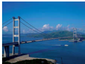
Tsing Ma Bridge, Hong Kong
