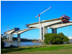
Gateway Bridge, Australia
