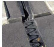
Cantilever finger joint
