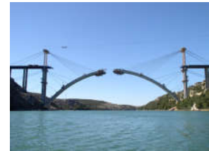
Krka Bridge, Croatia
