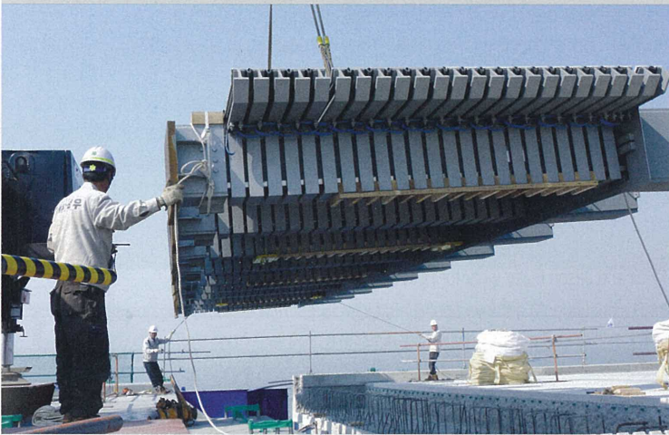
Above: The completed Incheon Grand Bridge (Amec) Above right: Transportation of joint from Austria to Hamburg by road Below: Installation of LR24 modular expansion joint on Incheon Grand Bridge
