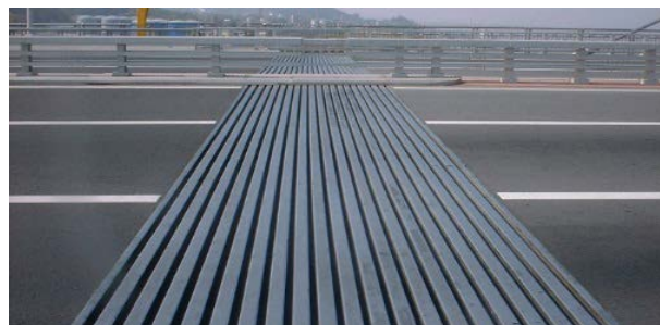
Figure 2. A modular expansion joint, viewed from above, showing the centerbeams and edgebeams that form its driving surface
