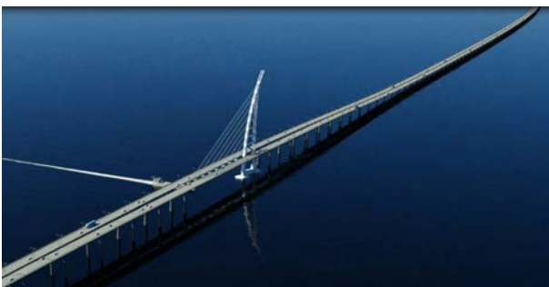
Figure 1. Artist's impression of the Sheikh Jaber Al-Ahmad Al-Sabah Causeway's main link, with length of 36 km, being constructed in Kuwait
