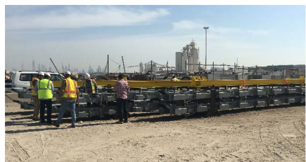
Figure 11. First modular expansion joints as delivered to site
