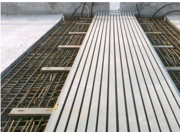
Figure 14. After the expansion joint has been precisely positioned, reinforcement can be placed around it as required in preparation for concreting
