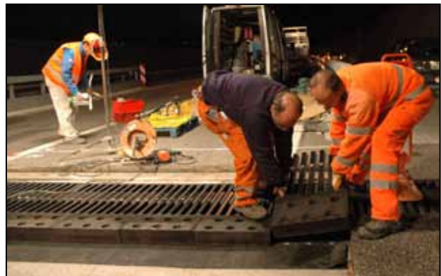
Fig. 10: Tensa® Flex Sliding finger joint (steel/elastomer bonded system) – during installation
