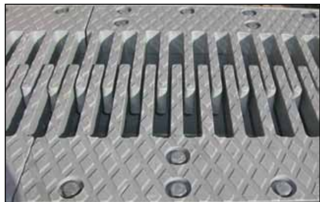
Fig. 8: Cantilever finger joint – as installed
