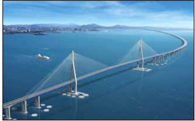
Fig. 13: The Incheon Bridge, South Korea
