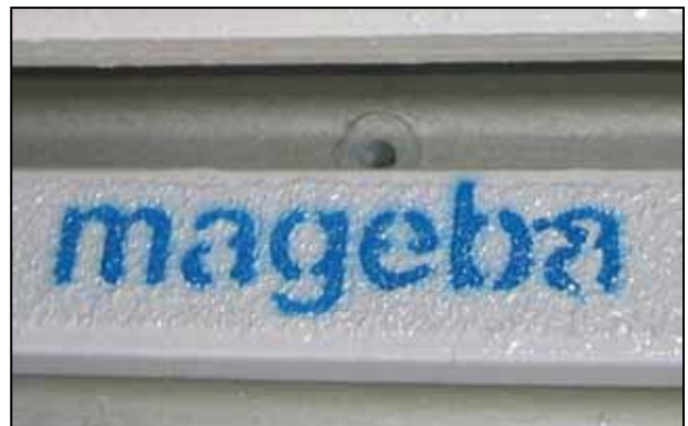
Fig. 5: Lamella surfaced with anti-skid coating
