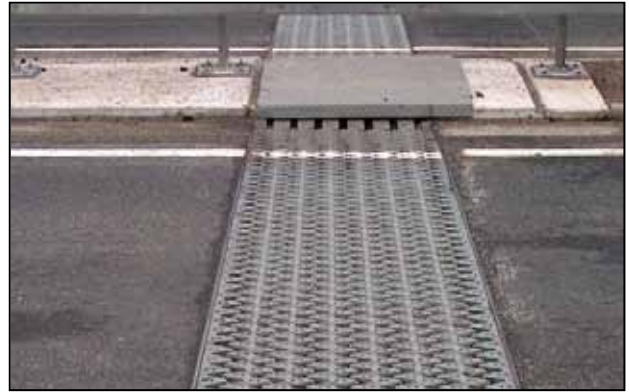
Fig. 4: Noise-reducing "sinus plates" on a modular joint
