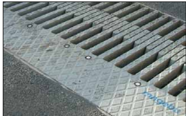
Figure 12. Sliding finger joint (steel system) – As – installed
