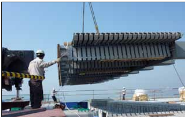
Fig. 16: Installation of a joint on the Incheon Grand Bridge, South Korea
