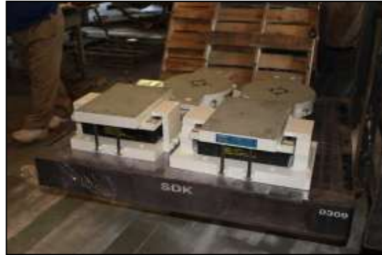
Figure 5. The bearings required by the bridge's design – including two uplift bearings at front.
