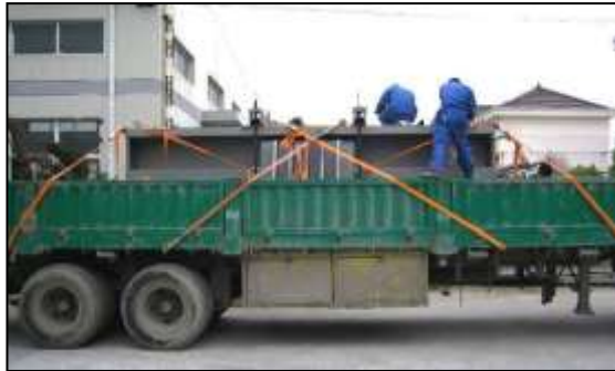
Figure 29. One bearing being secured on a truck for transport to site.
