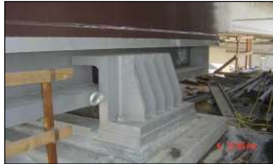
Figure 30. A bearing during installation on the Golden Ears Bridge.
