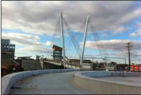
Figure 4. The new Revere Beach pedestrian bridge.
