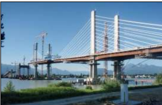
Figure 26. The Golden Ears Bridge, during construction
