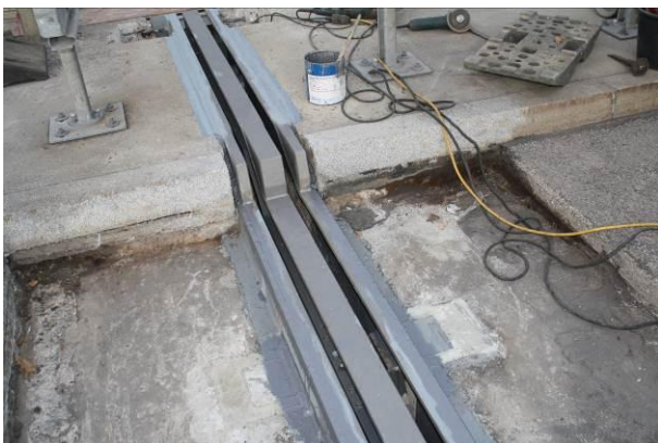
Fig. 17: Joint during application of corrosion protection
