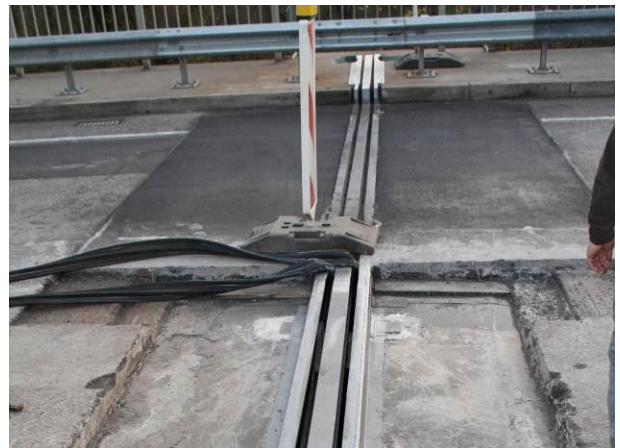
Fig. 22: View of joint following completion of first phase, before asphalt to finish second phase. The elastomeric sealing profiles (on left) have yet to be inserted in the second section
