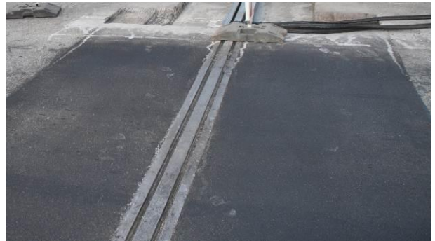
Fig. 20: Joint section following placing of asphalt at each side
