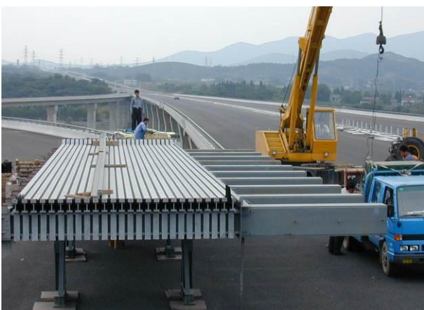
Fig. 2: A 27-gap modular joint prior to installation on the Run Yang Bridge, China
