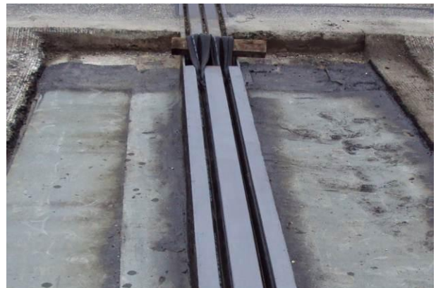
Fig. 18: Joint following insertion of sealing profiles
