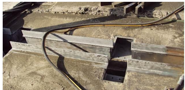
Fig. 10: View of the retained substructure following completion of cutting and removal
