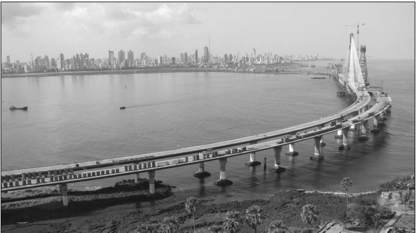
Figure 2. Bandra-Worli Sea Link during construction
