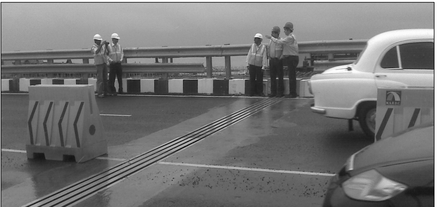
Figure 8 Installed modular expansion joint of the Bandra-Worli Sea Link
