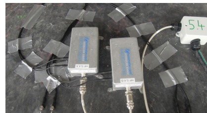
Humidity sensors installed on the underside of the roof
