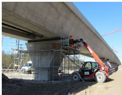
When a bridge bearing requires to be replaced, the costs (including for lifting of the bridge deck) can be substantial
