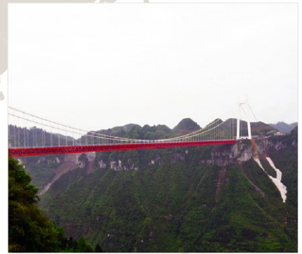
Aizhai Bridge | China
