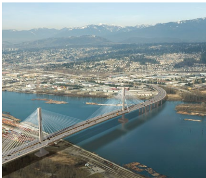
Port Mann Bridge | Canada
