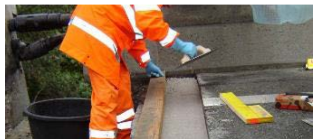
Figure 8. Robo®Flex support surface placed at each side of the joint for the Mini-Fly-Over plates, with dowels to secure them
