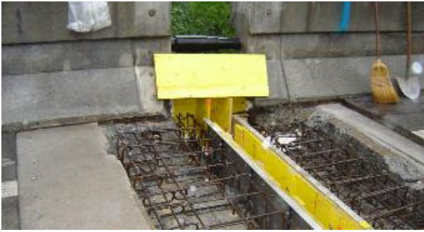
Figure 9. Robo®Flex support surfaces, dowels and shuttering in place
