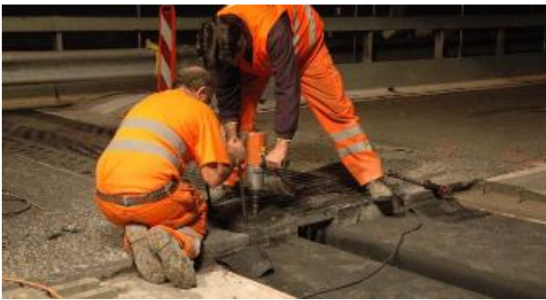
Figure 17. Finger plates anchored to dowels
