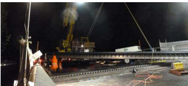
Figure 36. Lifting in of a new cantilever finger joint
