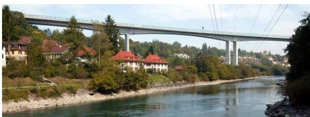
Figure 5. The Felsenau Viaduct, Berne
