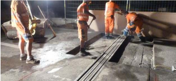
Figure 21. Removal of existing joint in first lane during first weekend
