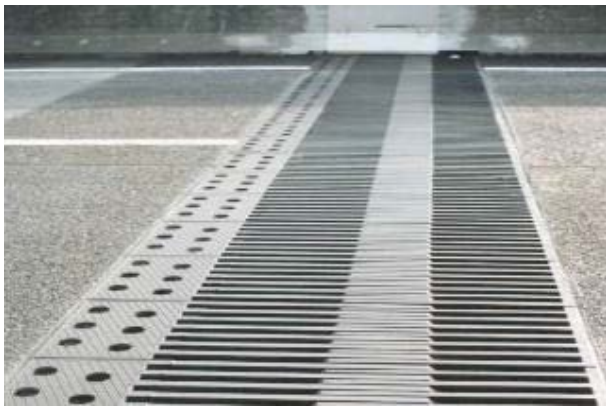
Figure 3. A Tensa®Flex expansion joint, as installed at the end of a road bridge
