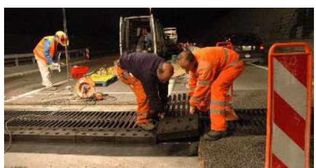
Figure 16. Tensa®Flex finger plates precisely positioned (by hand), element by element
