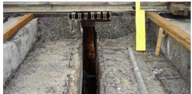
Figure 7. Recess cleanly excavated and subsoil compacted
