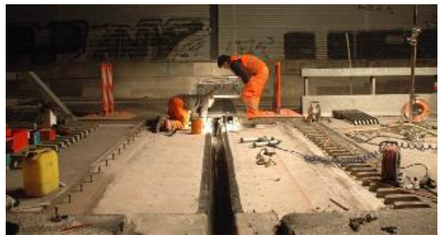
Figure 14. Drainage channel then placed and glued in position
