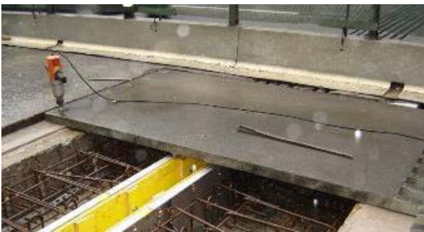
Figure 10. Mini-Fly-Over elements positioned and anchored in place at both sides of movement gap
