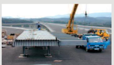
Design of Mageba's joints for the Runyang Bridge had to fulfil Certain requirements, including a design life of 50 years with design in accordance with BS5400, movement in all directions and rotational capacity about all three axes. The client wanted high durability of all components as well as the expansion joint as a whole, 100% water-tightness and low maintenance requirements, and easy exchangeability of all components.
