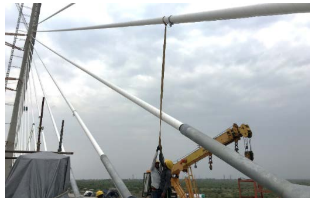
Figure 17. Forced vibration of stay cable with accelerometer during bridge construction phase
