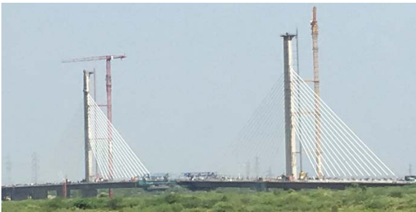
Figure 16. The Chambal Bridge during construction
