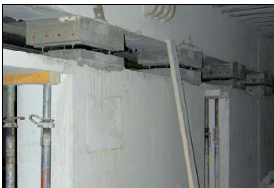
Figure 7. Sliding bearings inserted in internal basement wall
