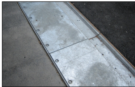
Figure 10. Installed expansion joint at vehicle exit
