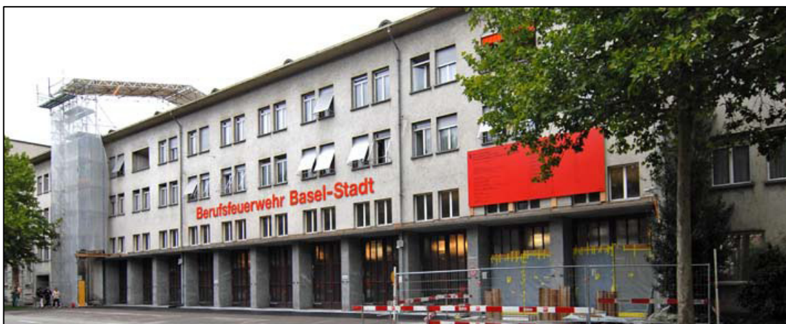
Figure 3. The central fire brigade building of the city of Basel, Switzerland
