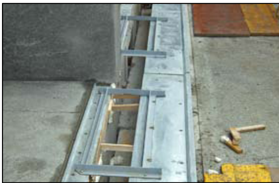
Figure 9. Installation of expansion joint
