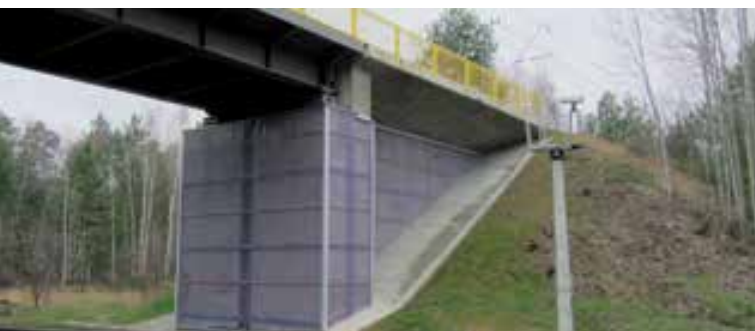
Abutment of the factory railway bridge, with added splash-water protection
