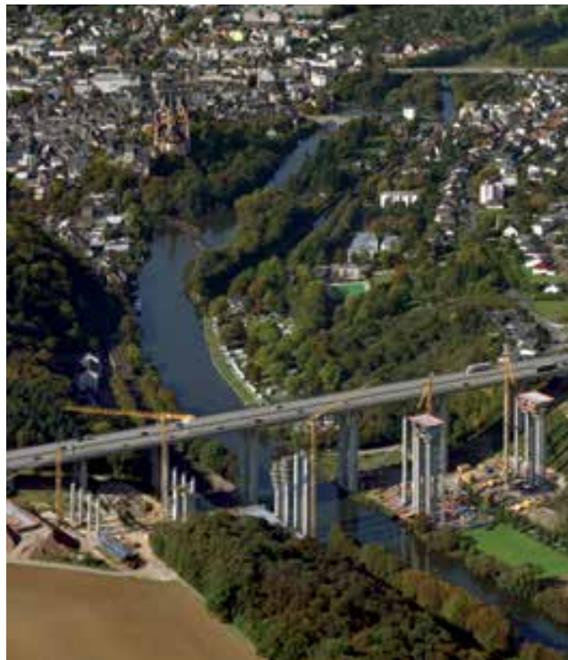
A3 autobahn, Lahntal Bridge, Nürnberg – Aerial photograph © Hajo Dietz
