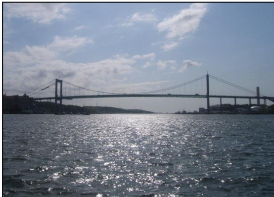
Figure 11. The Alvsborg Bridge in Gothenburg.
