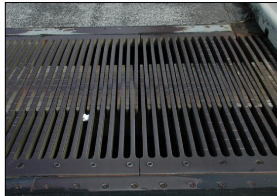
Figure 12. Existing finger joint of Alvsborg Bridge.
